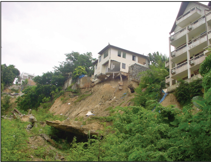
Figure 1: Na Nai roadside landslide events on October 25, 2007.
